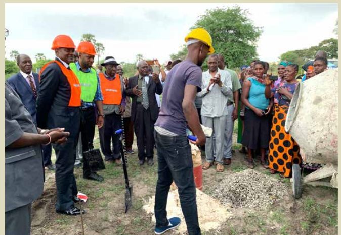
The ground-breaking ceremony was officiated by the Hon Pohamba Shifeta, Minister of Environment and Tourism on 24 November 2019 at Lusese Village, Kabbe South Constituency in Zambezi Region.
