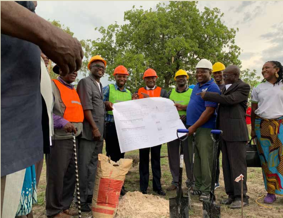
Hon. Pohamba Shifeta, Minister of Environment and Tourism officiating the groundbreaking ceremony at Lusese Village, Kabbe South Constituency in Zambezi Region.
